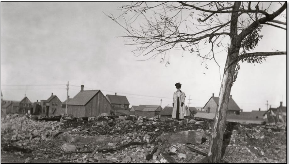
Figure 1: Ottawa–Hull fire of 1900
